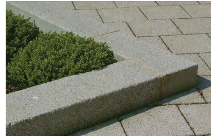
(6) Wide topped natural stone. Material: Silver grey granite flamed finish. Ebbsfleet Central, Villages Centres.
