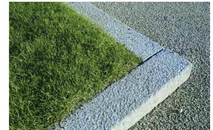
(8) Narrow topped natural stone. Material: Silver grey granite flamed finish. Level 3 & 4 Streets.
