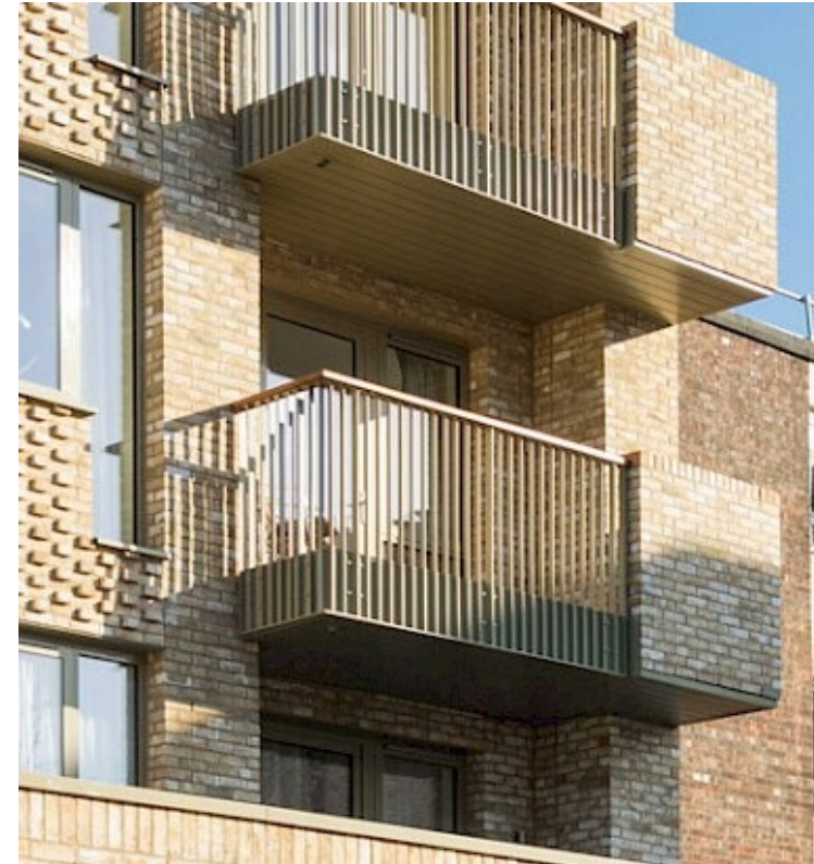
Hazelhurst Court, Beckenham Levitt Bernstein Architects
