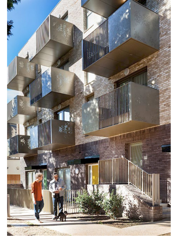
Dover Court, Islington Pollard Thomas Edwards Architects
