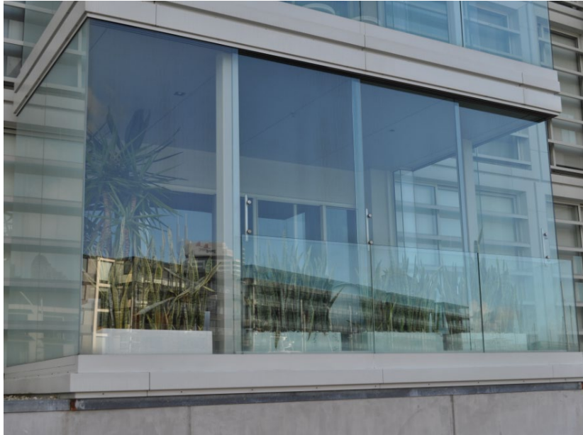
Lighter Quay, Auckland Studio Pacific Architects
