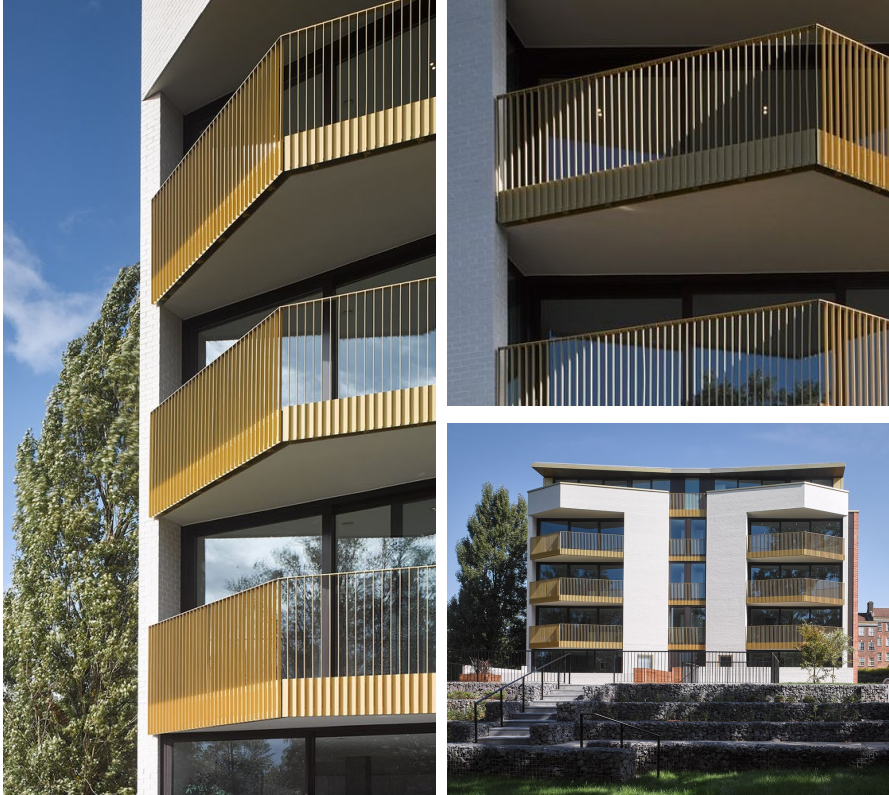
Bishopswood Court, Beckenham Daykin Marshall Architects
