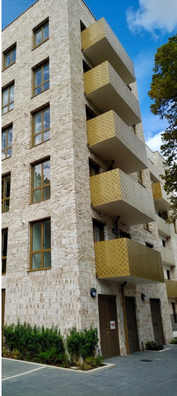
Regent's Park Estate Matthew Lloyd / Mae Architects
